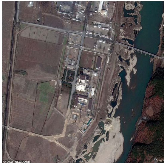
Construction at the North Korea's Yongbyon Nuclear complex in North Korea earlier this month
